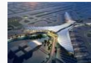
Expansion of King Abdulaziz International Airport, KSA
